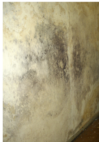
Figure 9: Black spot mould is a commonly associated with condensation. Photo: Douglas Kent
