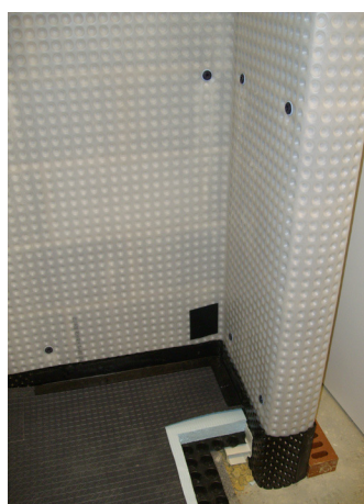
Figure 22: Ventilated dry linings can help with managing below-ground dampness where the underlying cause is difficult to address. Photo: Douglas Kent
