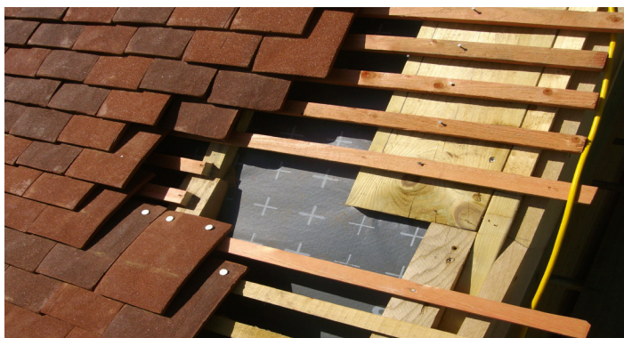
Figure 25: Manufacturers' instructions should be followed closely when installing vapour permeable membranes. Photo: Douglas Kent
