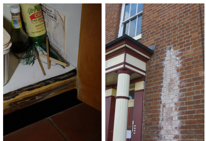
Figures 7(a) and 7(b): Plumbing leaks associated with: (a) Defective pipework above a kitchen unit (b) Overflowing WC cistern. Photos: Douglas Kent
