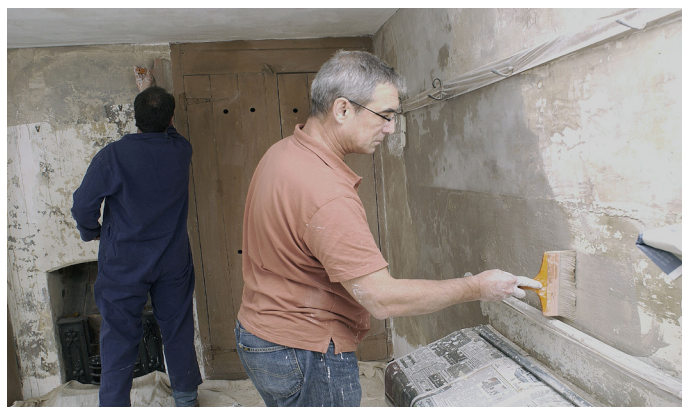
Figure 19: Vapour permeable paints, such as soft distemper, should be used when redecorating traditional solid walls. Photo: Douglas Kent
