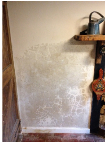
Figure 6: Rising dampness exists but is rarer than commonly supposed. Photo: Caroline Rye
