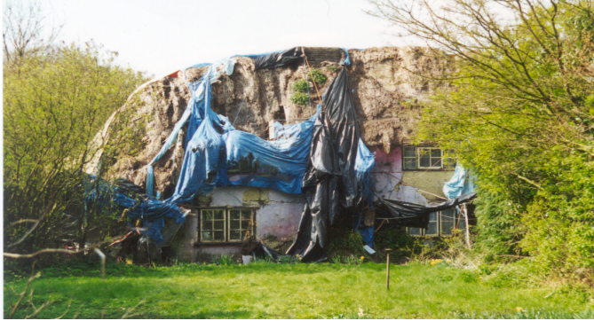
Figure 1: Dampness can lead to serious deterioration if left unattended, as with this cottage that was later demolished as a result. Photo: Douglas Kent
