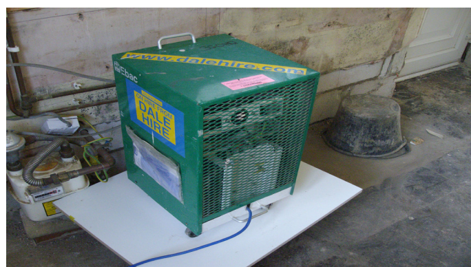
Figure 28: Dehumidifiers are rarely a practical long-term solution for condensation problems. Photo: Douglas Kent
