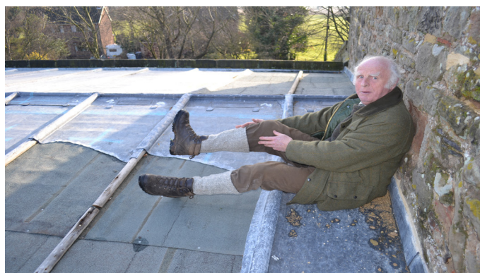
Figure 12(b): Damage from lead theft. Photo: Douglas Kent
