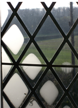
Figure 8: Condensation forms on the coldest surfaces first, such as windows or their surrounding reveals. Photo: Douglas Kent
