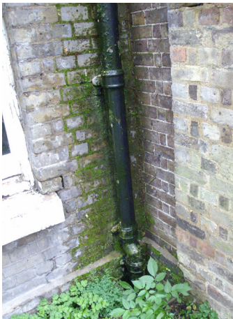
Figure 13: Moss growth can compound problems arising from rainwater penetration. Photo: Douglas Kent
