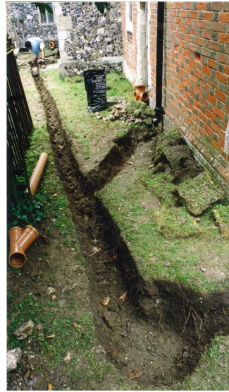
Figure 21: Improvements to drainage can help to overcome problems arising from below-ground dampness. Photo: Douglas Kent
