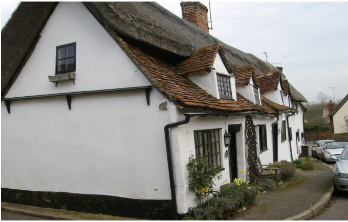
Figure 3: Traditional architectural details, such as pentice boards, function to protect buildings from the rain. Photograph: Douglas Kent
