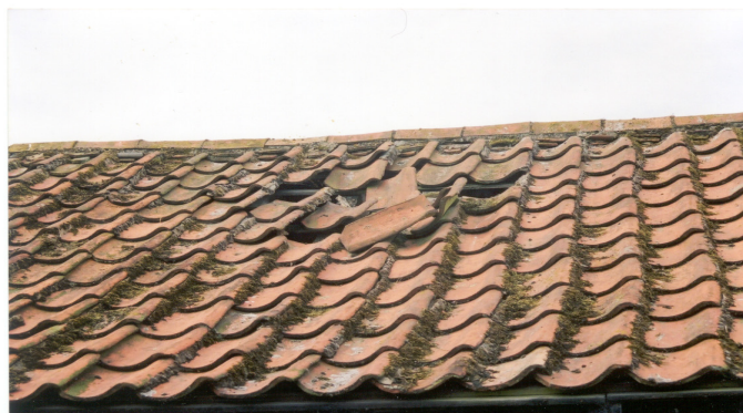
Figure 17: Diagnosis of a dampness problem is sometimes, but not always, obvious. Photo: Douglas Kent
