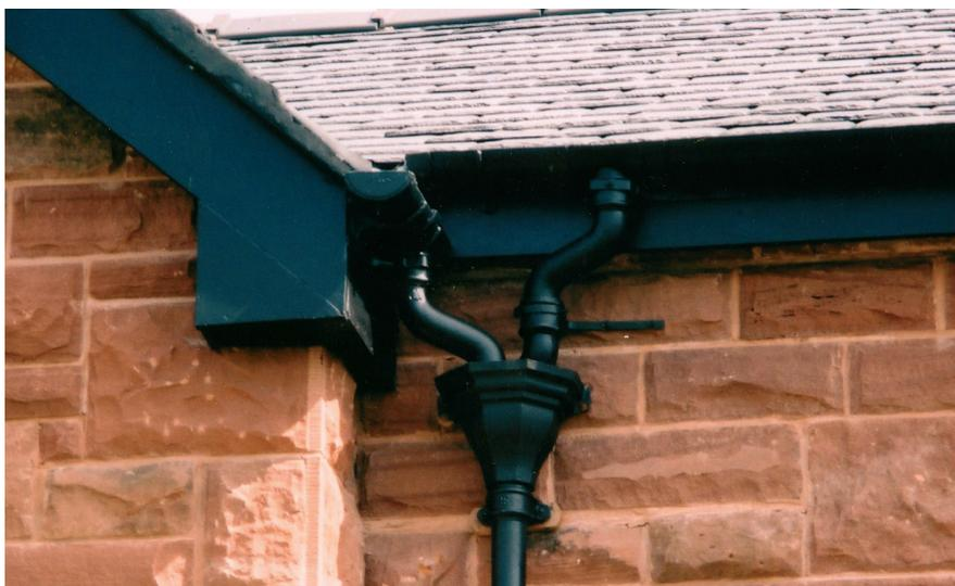
A reproduction of a typical late 19th century hopper with cast iron parapet gutters and simple ear bands on the down-pipe below
