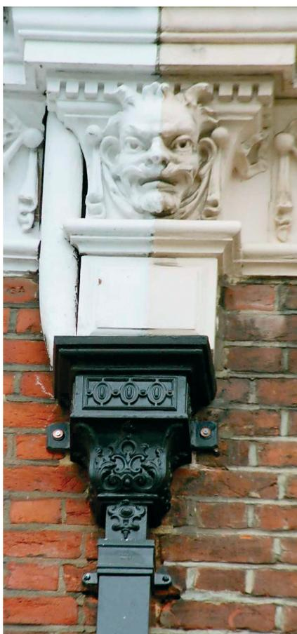
A particularly ornate early Victorian cast iron hopper head which collects water from a parapet gutter behind the fine timber fascia
